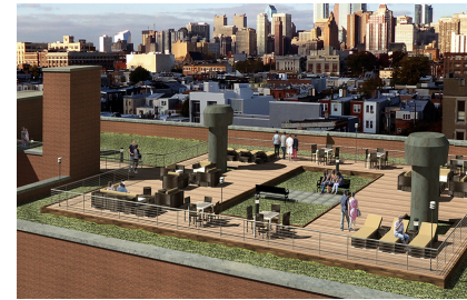
Green Roof Philadelphia
