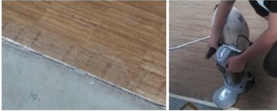
Grinding of the floor on the side with a corner grinder and level it with the middle floor
