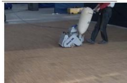
Horizontal grinding of floor
