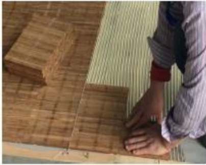
Glue two rows at a time and glue with 1/2 board
