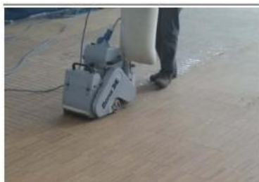
Vertical grinding of floors
